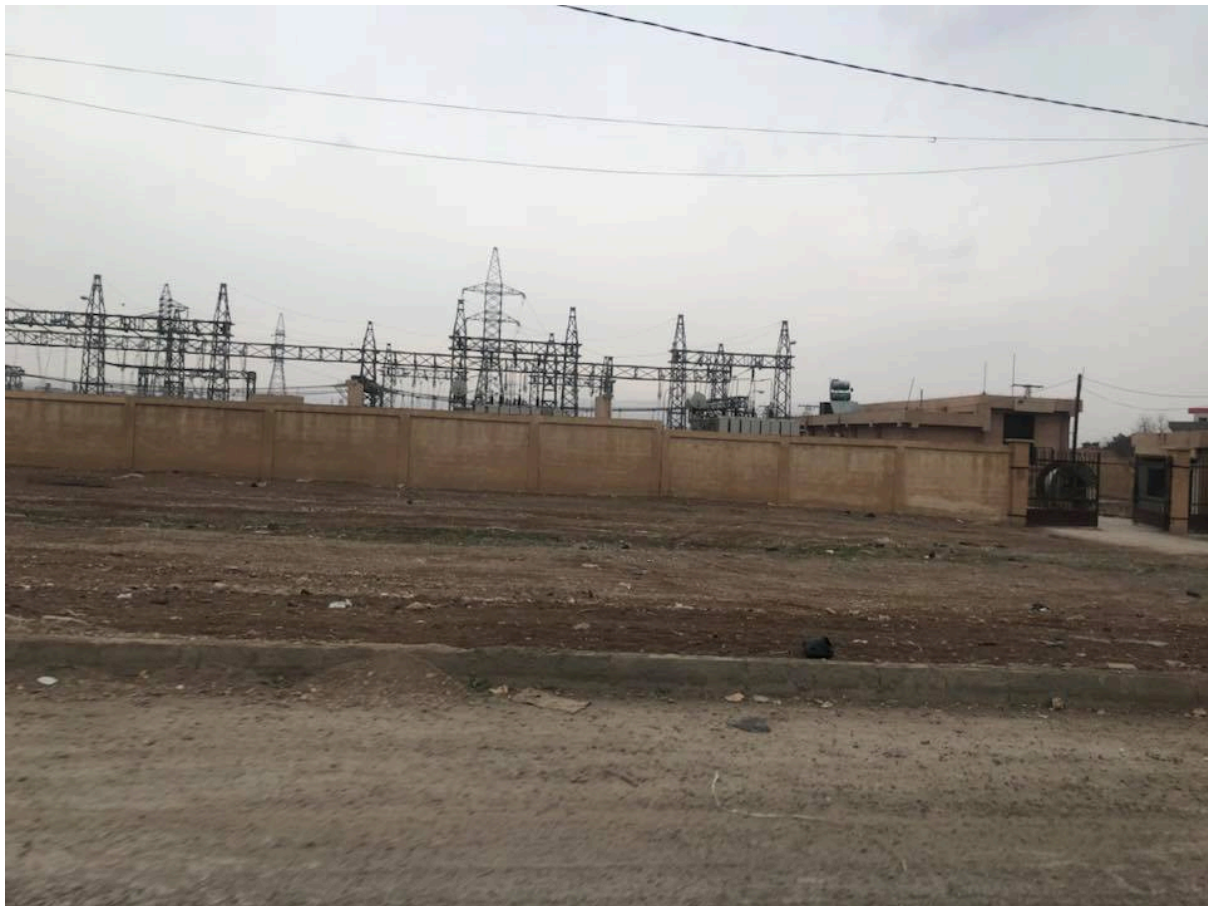
Outside the regime-affiliated electricity station and office in Qamishli
